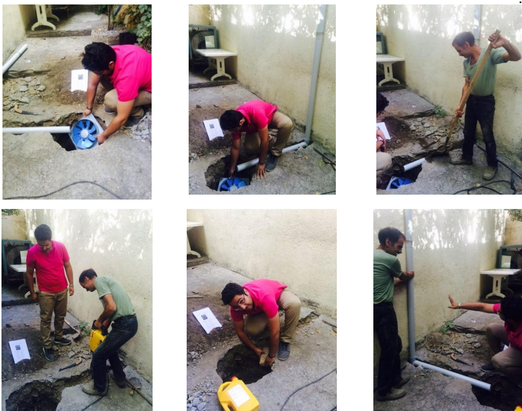
Figure 1 Appendix: Implementation of Radon gas reduction project in a sample building in the Kohe-Sangi of Mashhad
